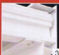
Wall plate fixed to wall
